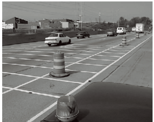
Rumble strip for work zone speed control
