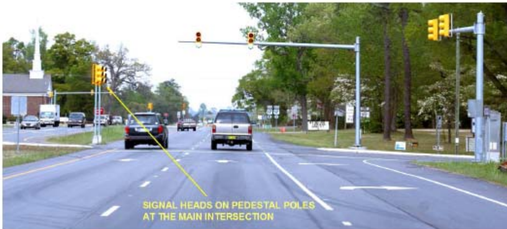
Figure 28: Signal Pole Locations at an RCI on US-17 in North Carolina
