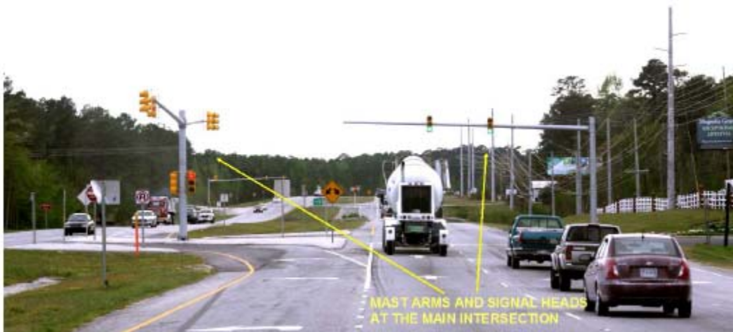
Figure 27: Signal Pole Locations at an RCI on US-17 in North Carolina
