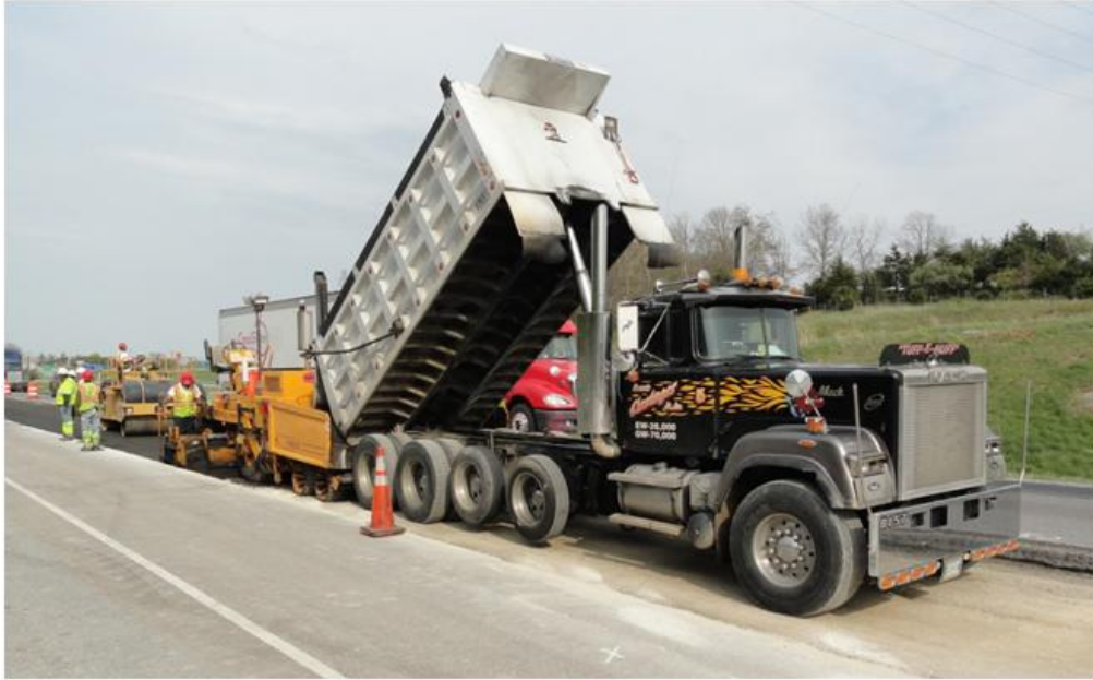
Figure 5. Paving the Cold Central-Plant Recycling Material
