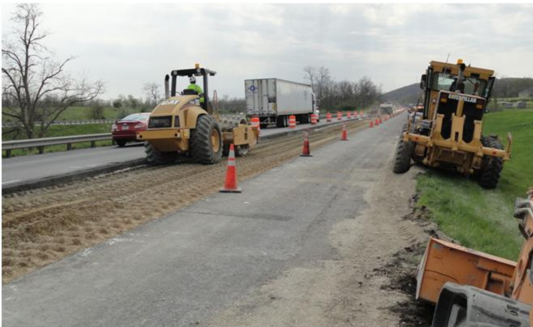
Figure 3. Compaction of Full-Depth Reclamation Layer
